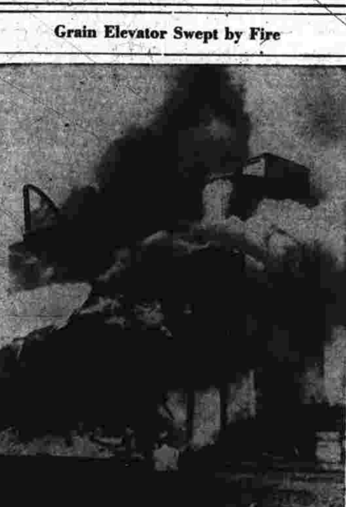
Grain Elevator Swept by Fire
